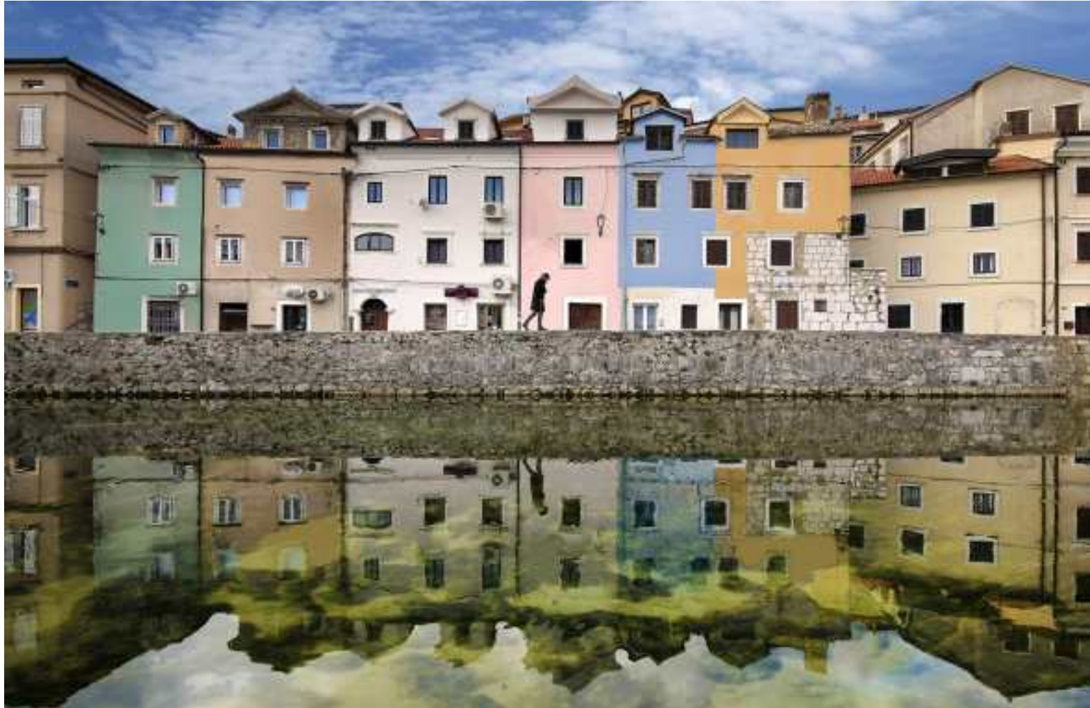
Promenade At The Coper City
